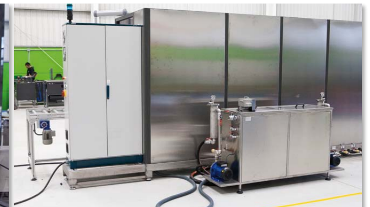
Decanting of oils and filtration tanks.
